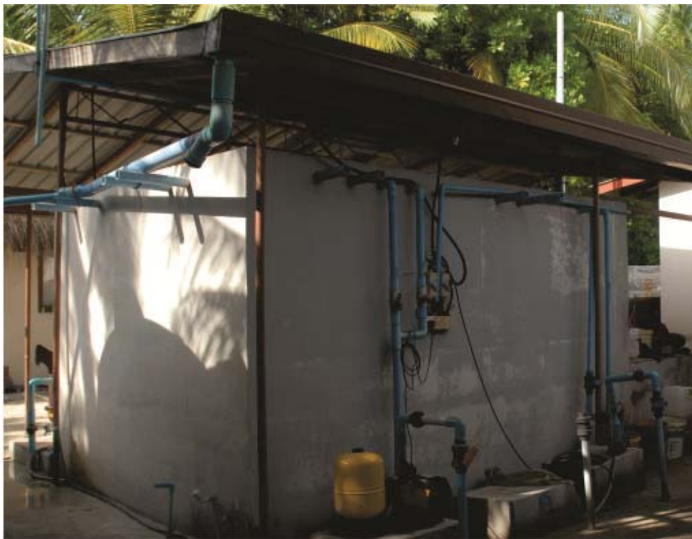
Figure 1: Sedimentation tank
