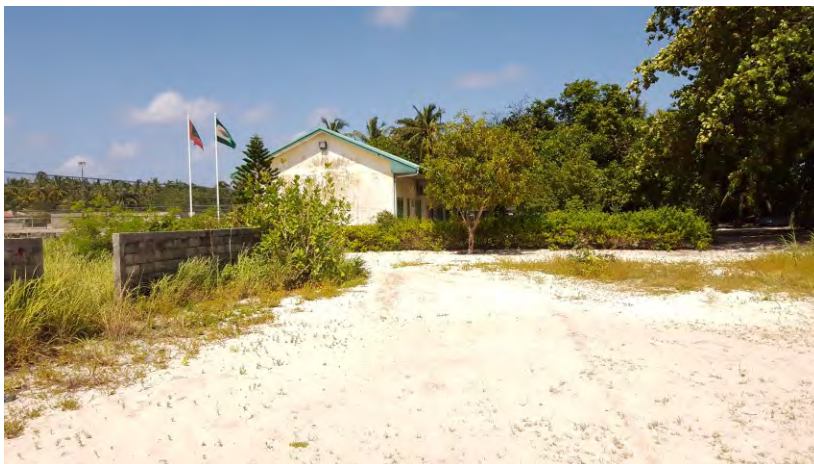
Figure 4.16: The existing FENAKA site opposite to the proposed RO plant site
