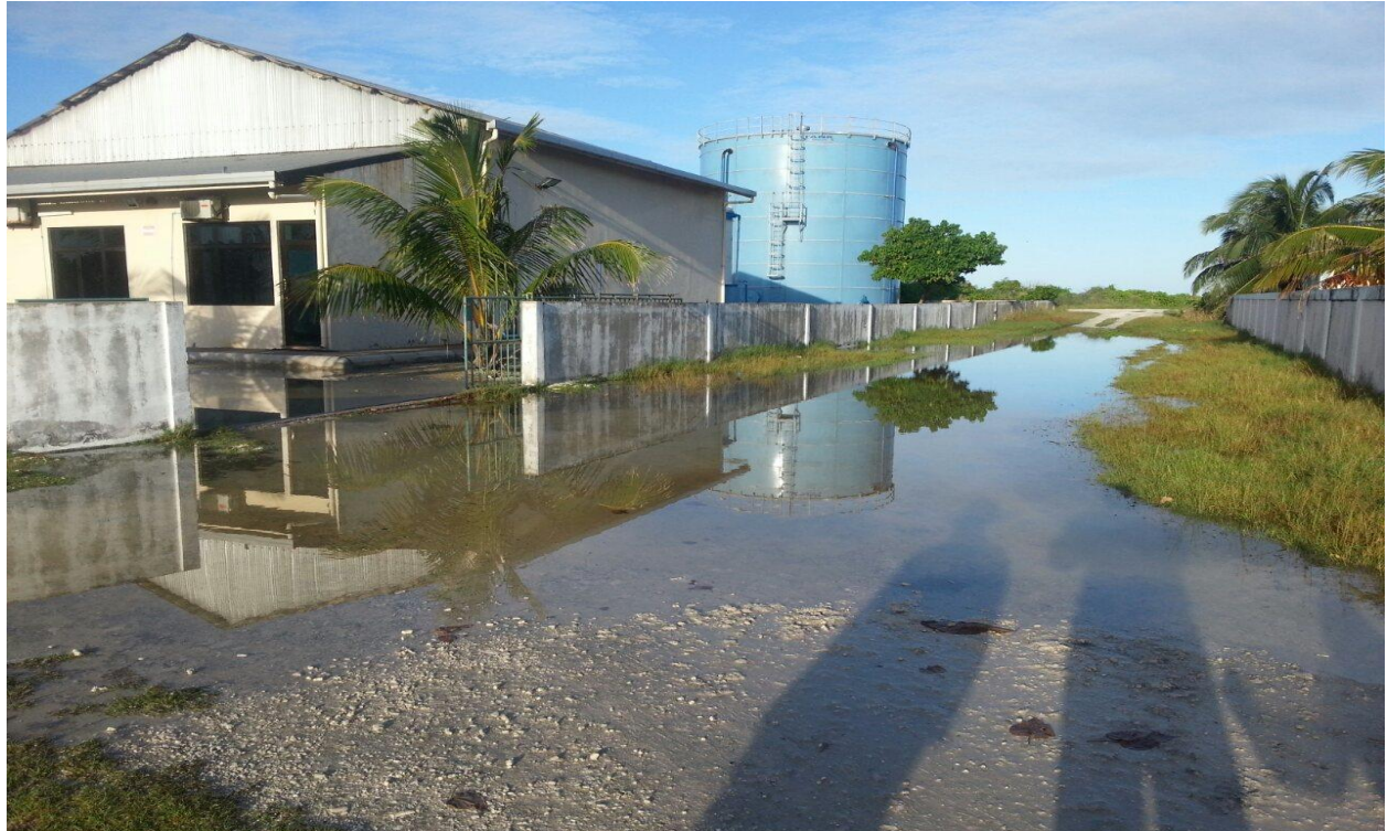
Figure 19: flooding during rainy season at powerhouse area
