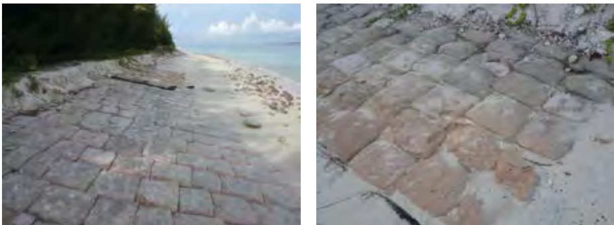
Figure 4.24 Generic revetment design – Sand-cement bags in Hulhumale'
