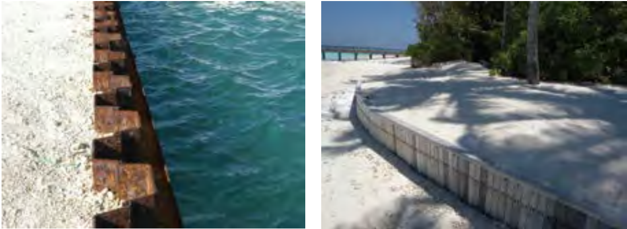
Figure 4.9 Examples of Seawall structures: unplastered sand cement bag seawall in M. Maduvvari and Sun Island Resort
