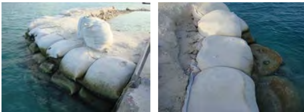
Figure 4.14 Adhoc seawalls in (clockwise from left) GA. Dhevvdhoo , GDH Thinadhoo, GA Kolamaafushi and B. Eydhafushi
