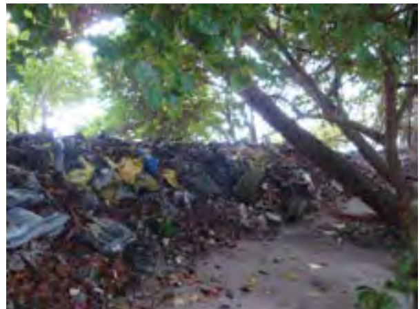
Figure 5.20 Use of both construction debris and green waste as an adaptation measure against erosion in HDh. Hanimaadhoo and V. Keyodhoo
