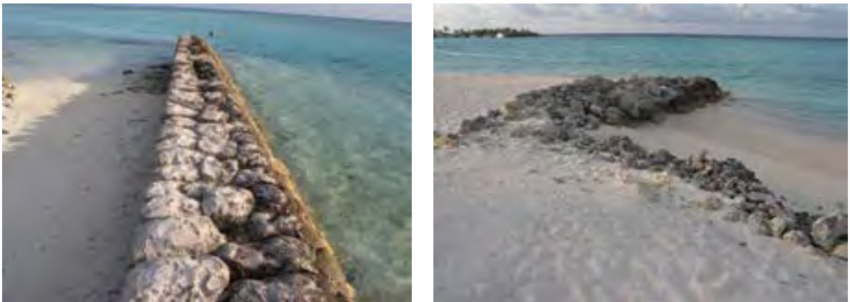
Figure 4.29 Groynes constructed from coral rubble in B. Reethi beach and AA Bodufolhudhoo
