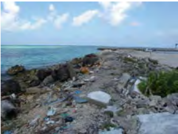
Figure 5.20 Use of both construction debris and green waste as an adaptation measure against erosion in HDh. Hanimaadhoo and V. Keyodhoo
