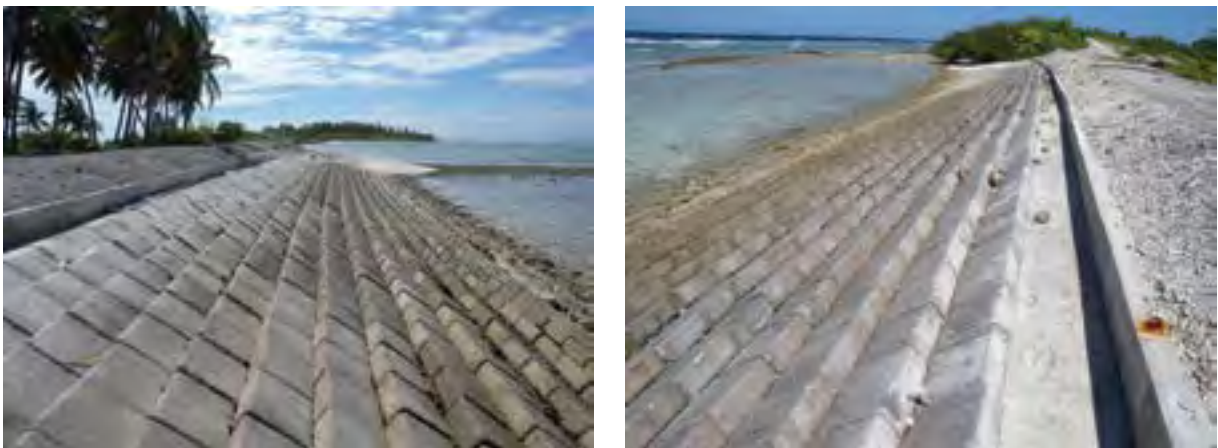
Figure 4.24 Generic revetment design – Sand-cement bags in Hulhumale'
