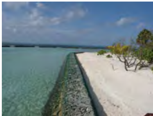
Figure 4.8 Examples of Seawall structures: unplastered coral mound seawalls in M. Maduvvari and Lh.
