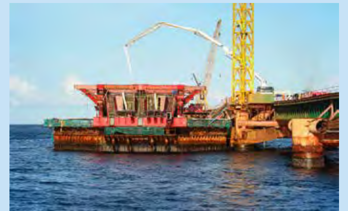
The arch legs shaped like a V started off from the pier cap. This photo is dated 3 rd August 2017. 2017年8月3日，中马友谊大桥主桥19#墩V墩第一节段混凝土浇筑
