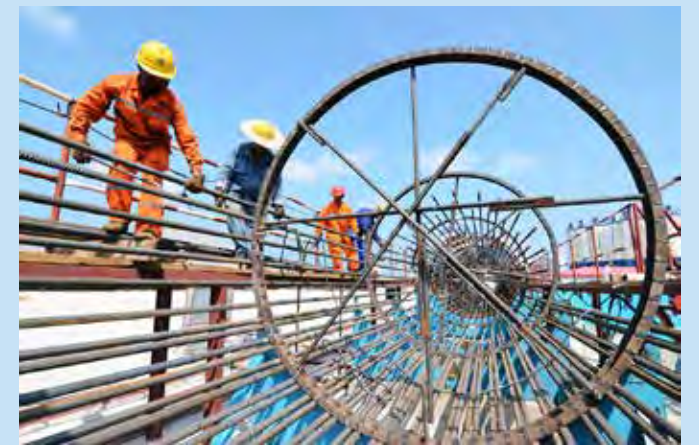
The reinforcement cages for the large piles are necessarily large. The photos show cages being made ashore.
