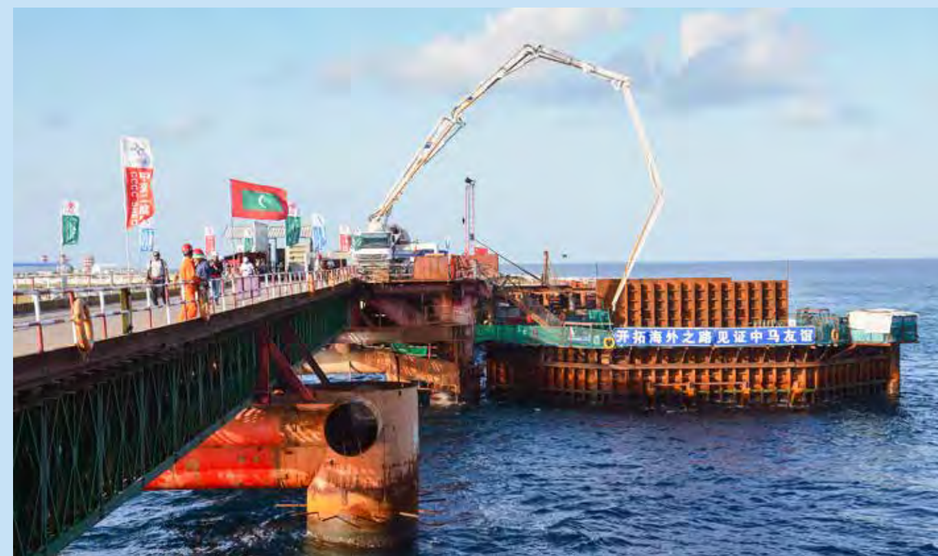
These photos show the middle pier of the bridge. Once the cofferdam was completed, pouring concrete into it started on 13 th May 2017 (above). Pouring was completed on 20 th July 2017 (below).
