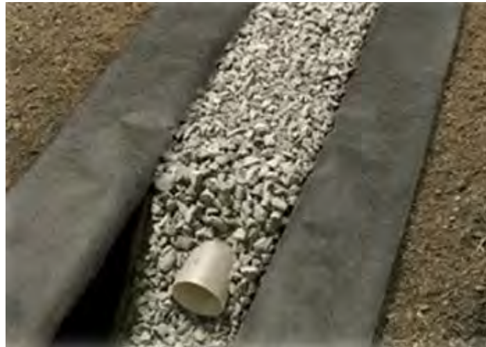
Figure 2.21: Typical section through a road filter drain (CIRIA, 2015, p. 149)
