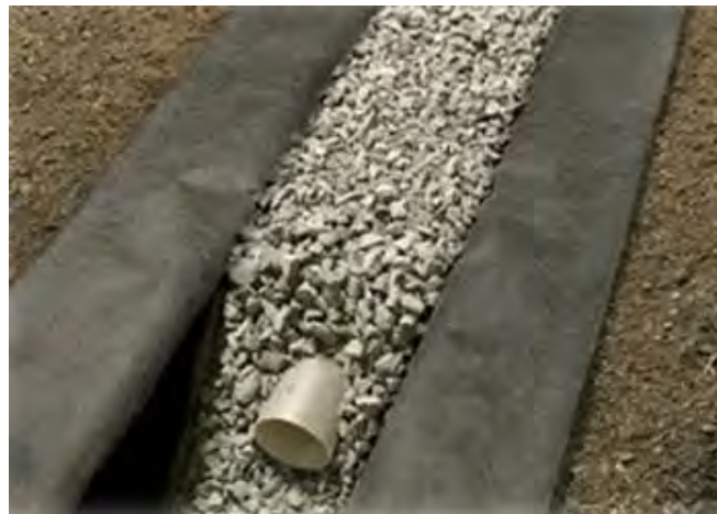
Figure 1.9: A filter drain under construction (Source: edensstructural.com)
