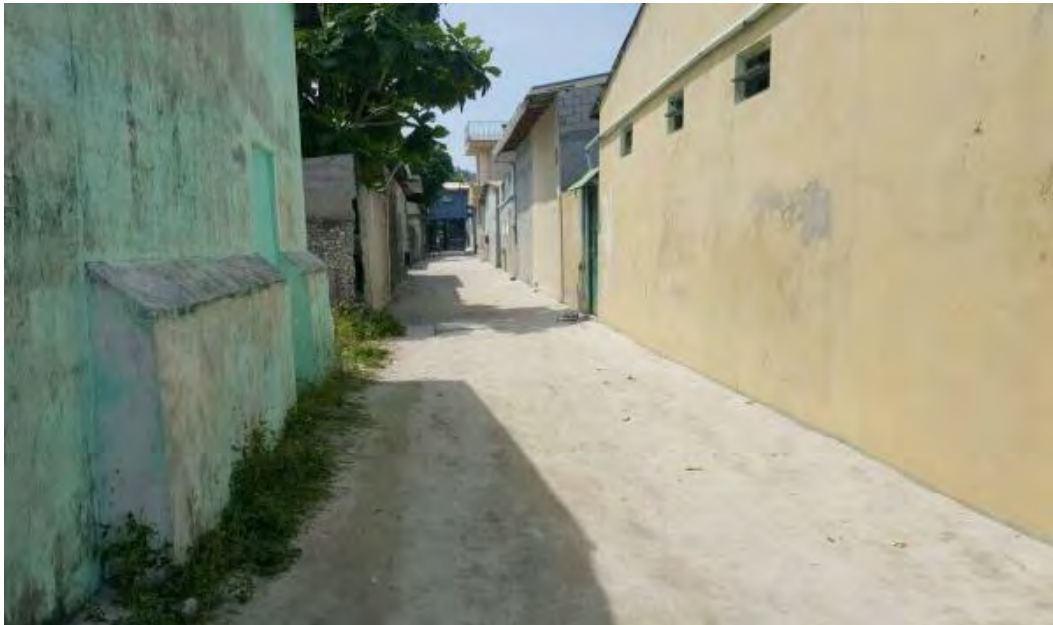
Figure 4: Surface runoff will infiltrate into the groundwater through sandy soil in the islands (Shown here is a typical unpaved sandy road in an island) (Source: raajje.mv/4062)
