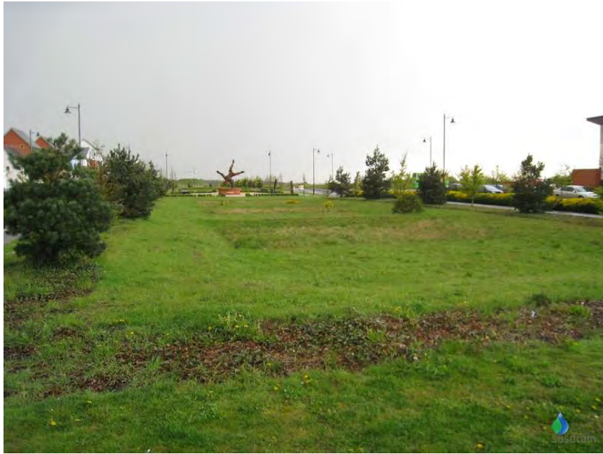
Figure 2.17: Picture of an infiltration basin, in dry condition (Source: susdrain.org)
