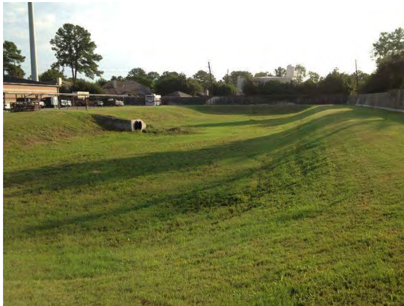
Figure 1.12: Example of a large infiltration basin suitable for areas with plenty of open free space (Source: cityofoberlin.com)
