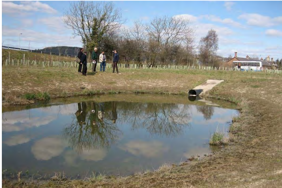
Figure 2.18: An example of a retention basin (Source: abertay.ac.uk/business/facilities-and-services-2020/SuDSnet/SuDSnet-photos/retention-ponds/ )
