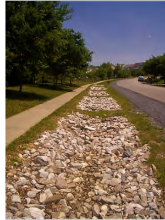
Figure 1.8: Cross-section through an infiltration trench (left). Example photo of an infiltration trench constructed on the road side(right) (Adapted from Source: sswm.info)
