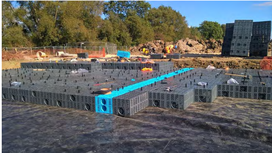
Figure 2.25: Geocellular tank units are being installed in a park (Source: blog.wavin.co.uk )
