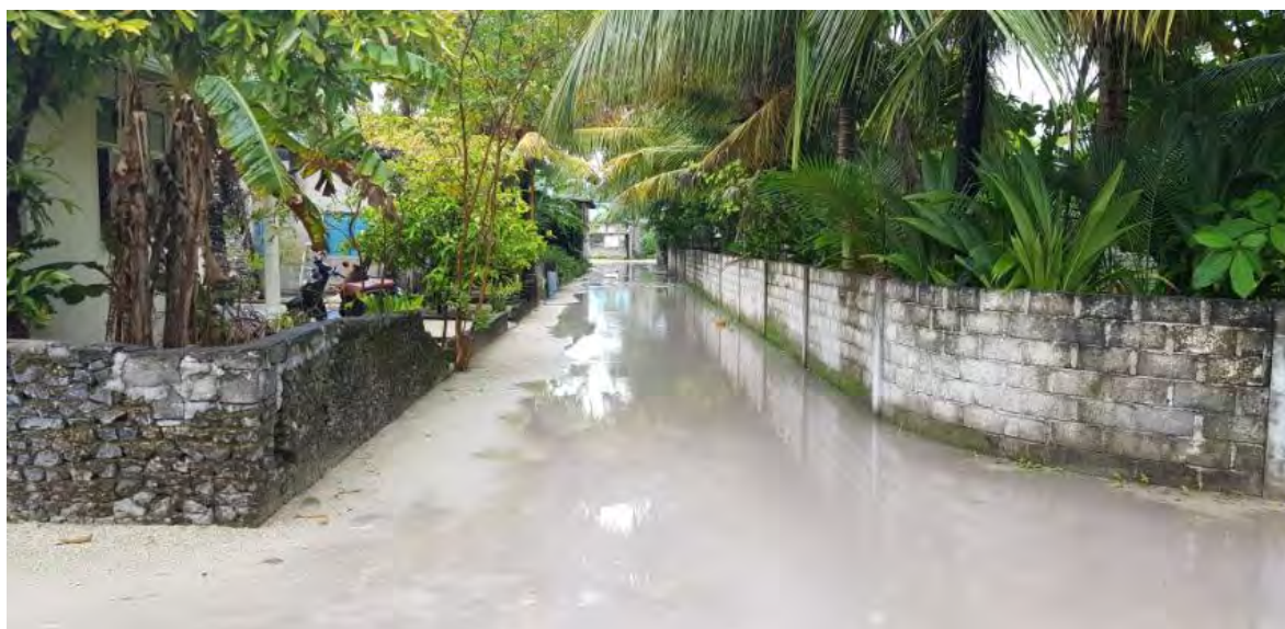
Figure 2.3: Ponding and flooding observed on the surface of an unpaved road in Ga. Maamendhoo after a rainfall event (Source: Authors)
