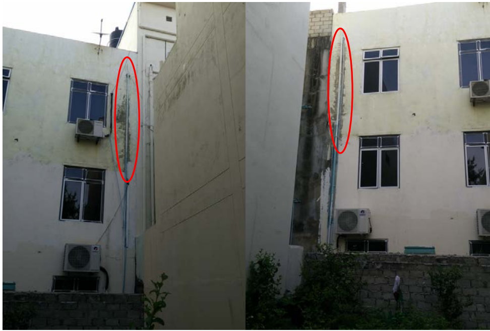
Figure 11: Entrance to the building in lot 10090 at Nirolhumagu (top) back of the building showing the condition of wall and water leakage
