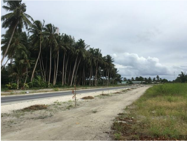
Figure 4.13: The newly developed link road adjacent to the RO Plant Site
