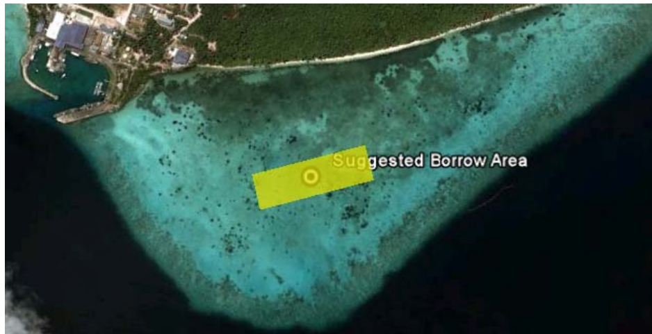
Figure 7: Suggested borrow area for material for the base-layers of the air-field. Also see Annex 4.
