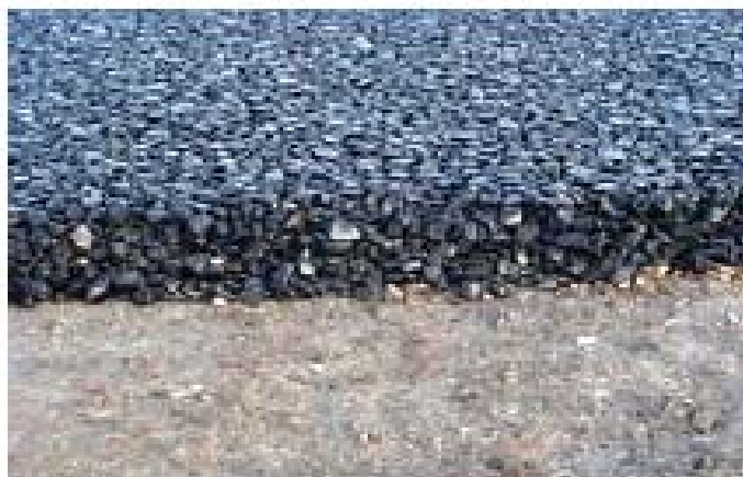
Figure 6: Rock aggregate base layers (bottom) with porous asphalt layer on top required for the air-field. Image extracted from Naeem et. al, 2008.
