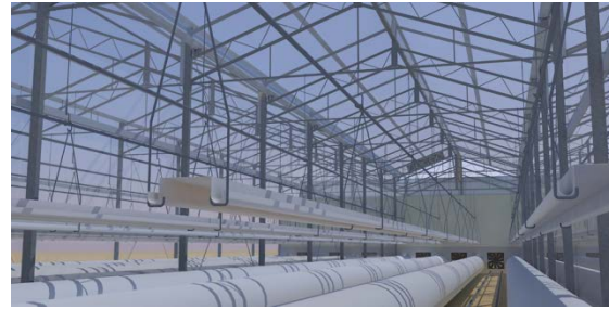
Hanging gutters where the plants will be hosted
