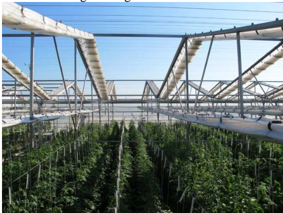
Greenhouse completely set up
