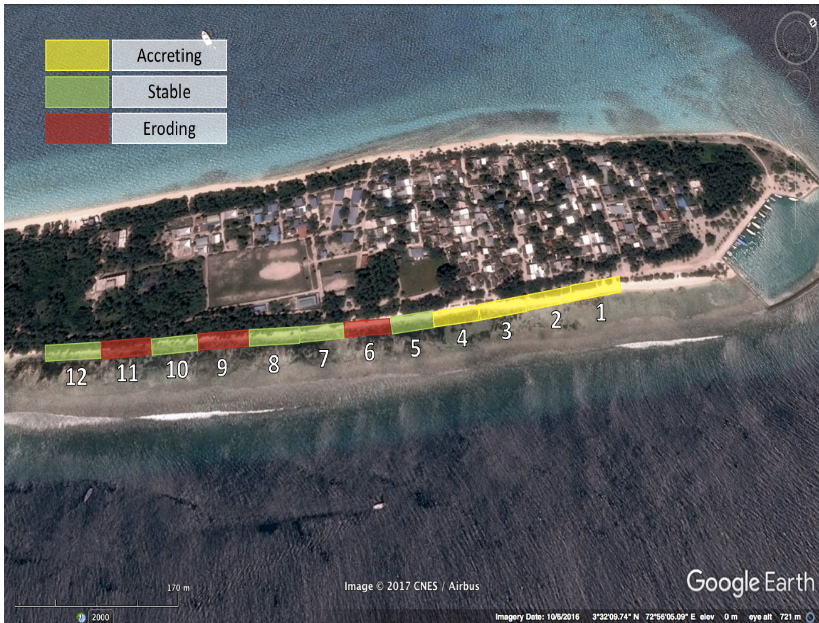
Figure 6.12: Google Earth image with the results of the shoreline stability survey at sites 1 – 12.
