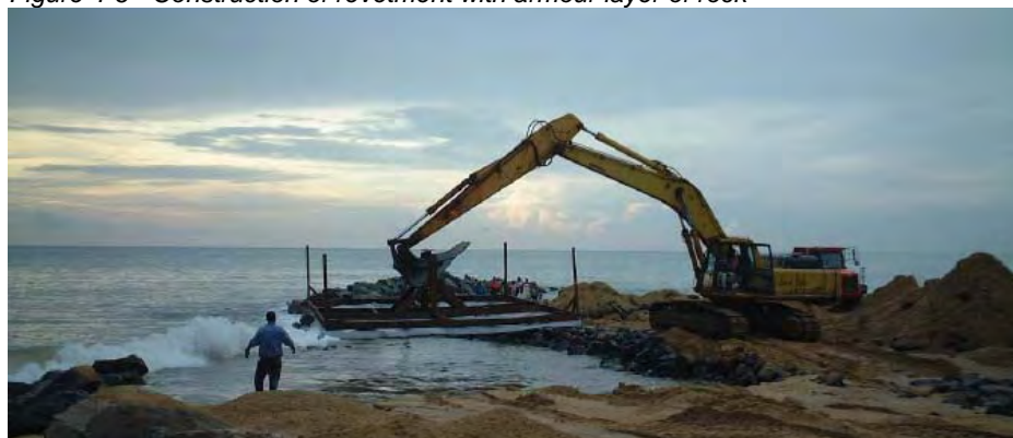
Figure 4-6 - Construction of revetment with armour layer of rock
