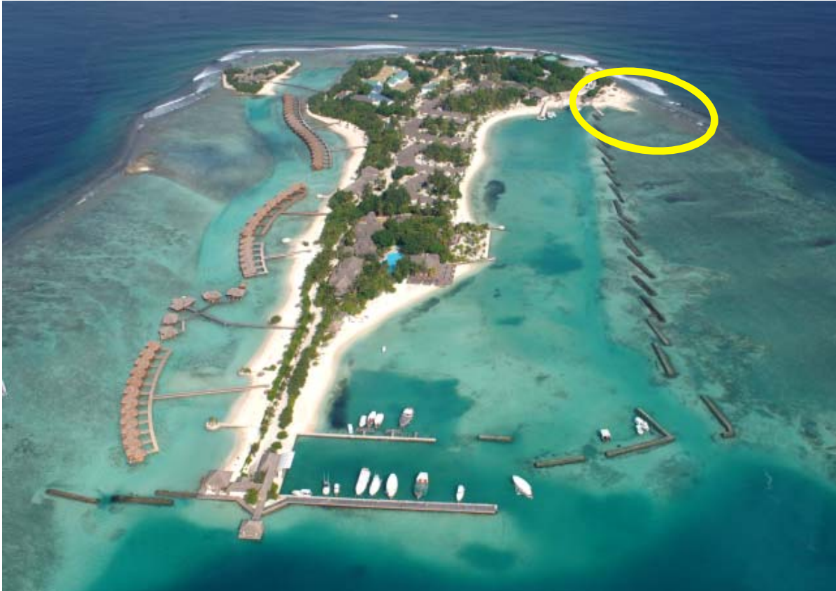
Figure 1: Over view of Fullmoon resort looking from western side towards east. The main features of the Fullmoon Resort – the breakwaters are seen. The circled area is the project area.
