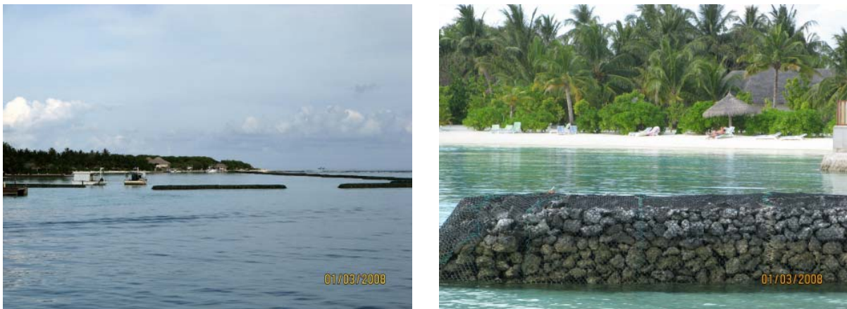
Figure 10: The beach on the southern side (right) is maintained regular 'beach replenishment' using 2 sand pumps (right) which are placed in the lagoon.
