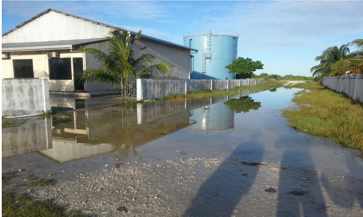
Figure 17: flooding during rainy season at powerhouse area
