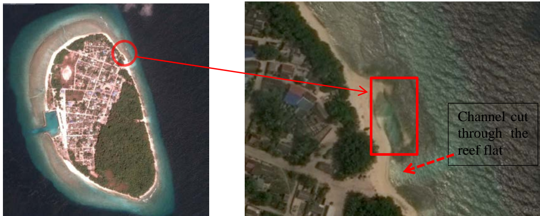
Figure 3: Alternative access channel and dredged area developed in 2011, soon became filled with sand and rubble.
