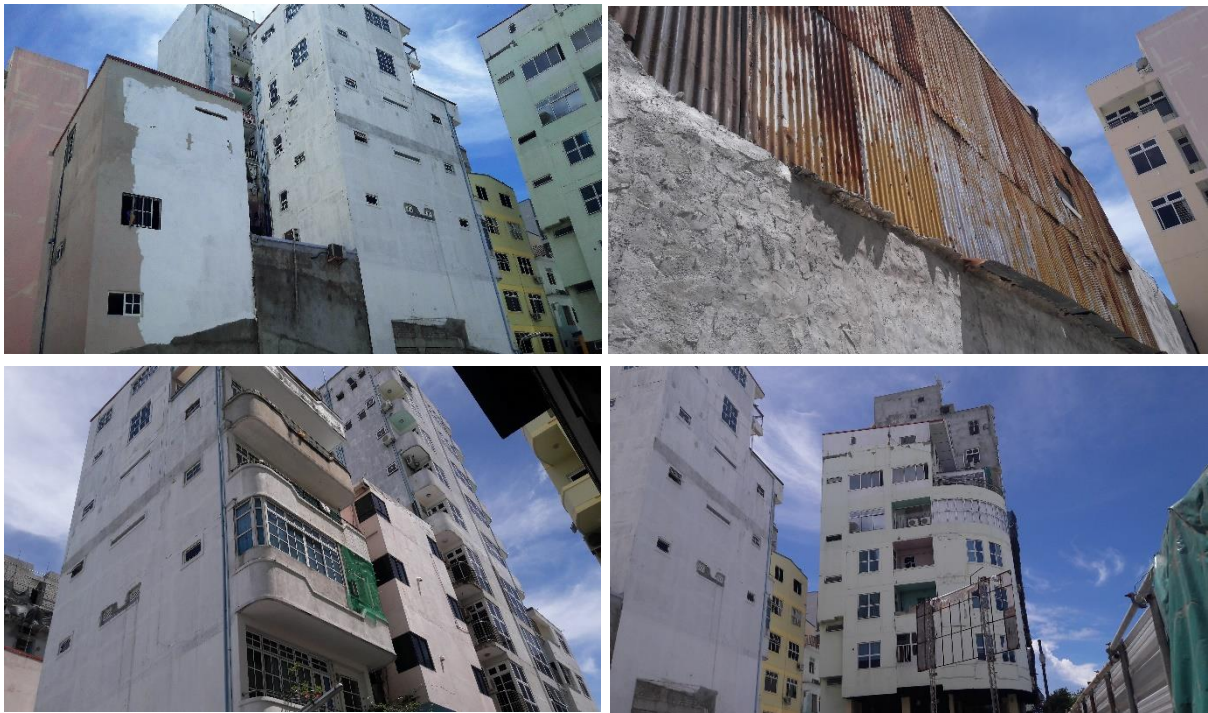
Figure 32: Condition of the buildings by the plot and opposite
