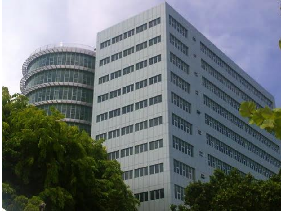
Figure 6: The 14 Storey Velaanaage Office Complex
