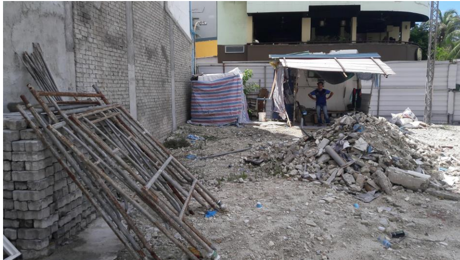
Figure 8: Temporary security hut and fencing within the plot
