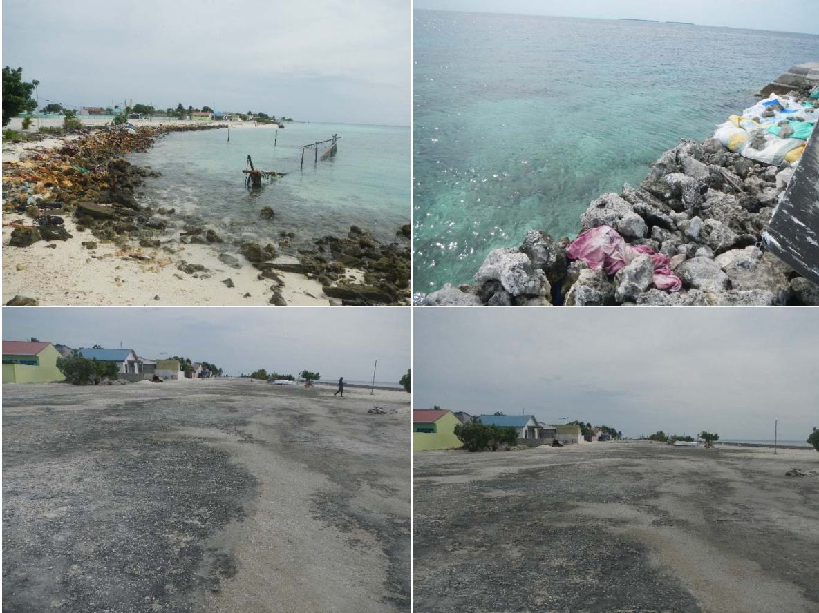
Figure 5: Condition of the places where the construct material will be deposited (above) and the road conditions (below).
