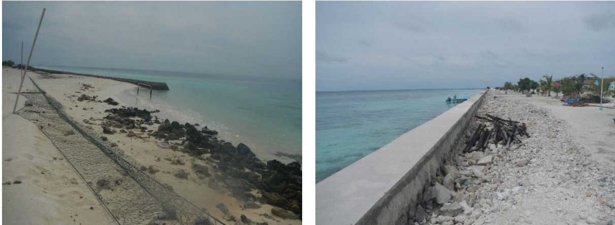
Figure 13: Coastal environment of (left) where the new quay wall would be constructed and (right) where the land would be reclaimed.
