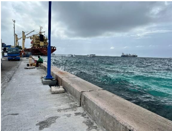
Figure 6.2: Off-loading area in the main port which is flood-prone
