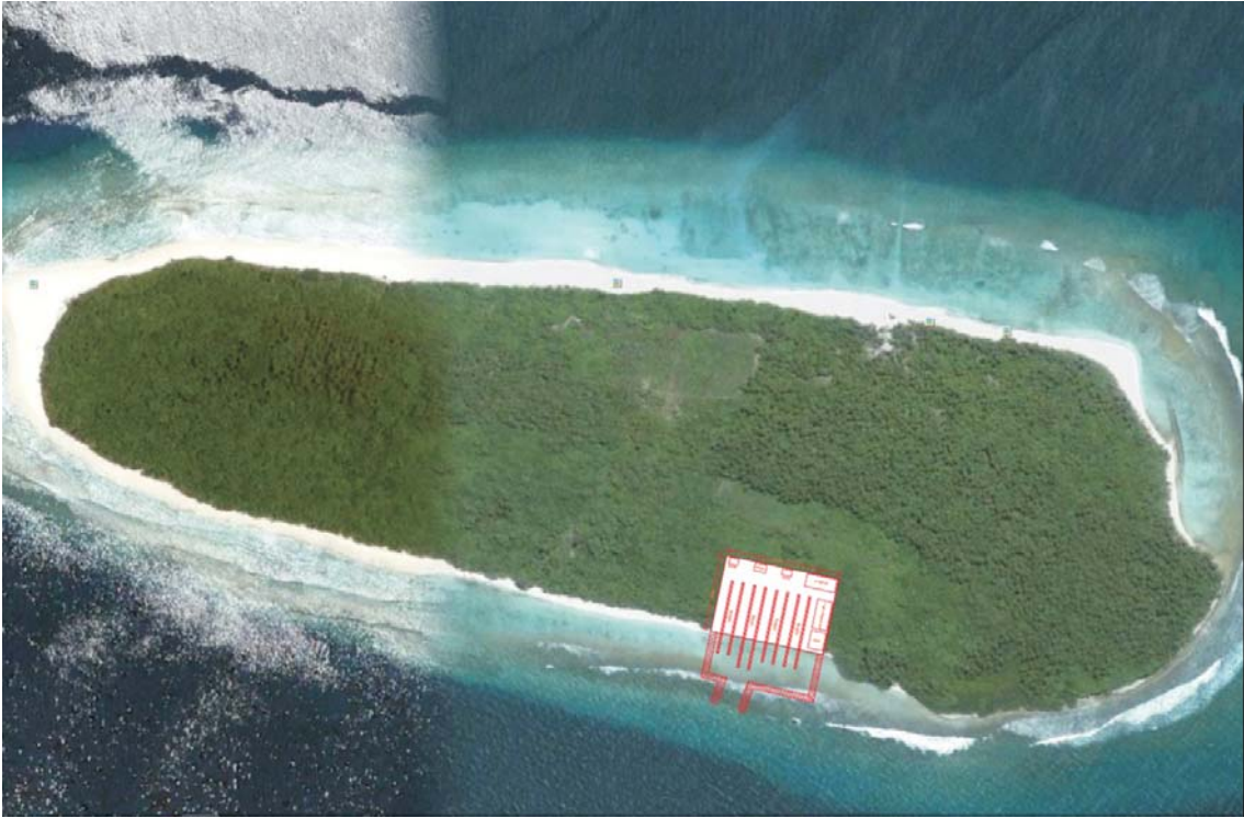
Figure 1: Location of the Slipway.
