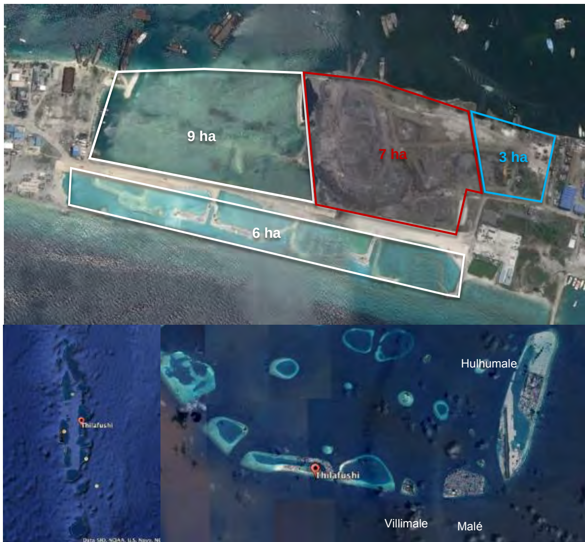
Figure 1: Thilafushi Island and current dumpsite (red, upper picture), white-rimmed plot is the envisaged area for the RWMF (source: Google Earth).
