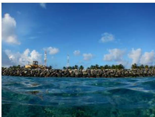
Figure 4.28: Rock boulders protecting the shoreline at the site
