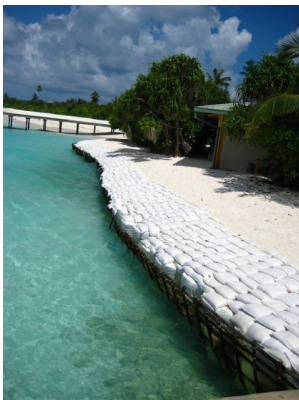
Figure 14. Sea wall of sand cement bags
