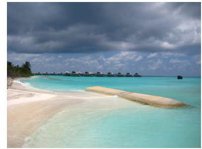
Figure 13. Geotubes installed by Seamarc
