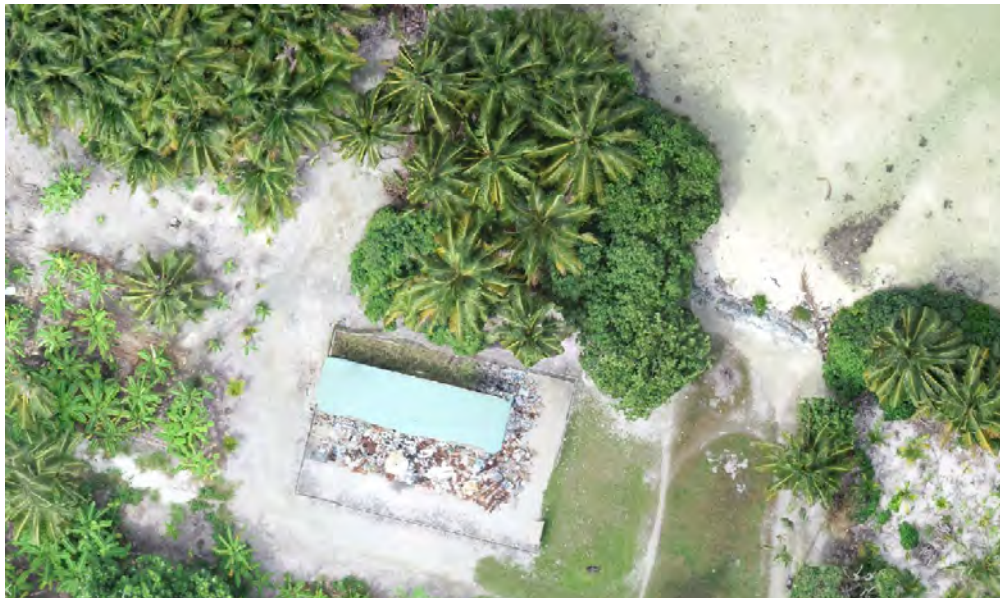
Figure 9. Drone image of existing WMC: the structure is very close to shoreline and does not meet the EPA guidelines of 30m offset from vegetation line
