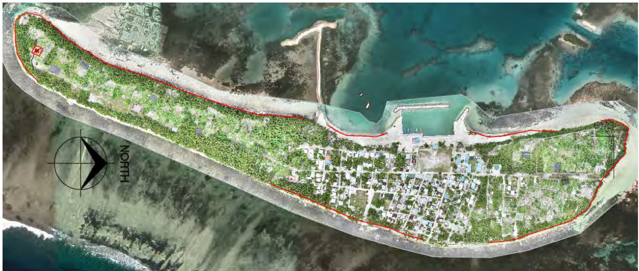
Figure 12. Erosion areas at Dhanbidhoo (red lines at shoreline)
