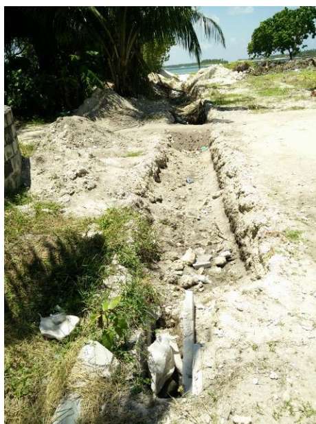
Figure 6: tranches made to drain flood water
