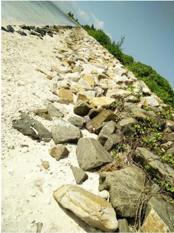
Figure 8: existing beach and rock boulder revetment on the eastern side of Villingili
