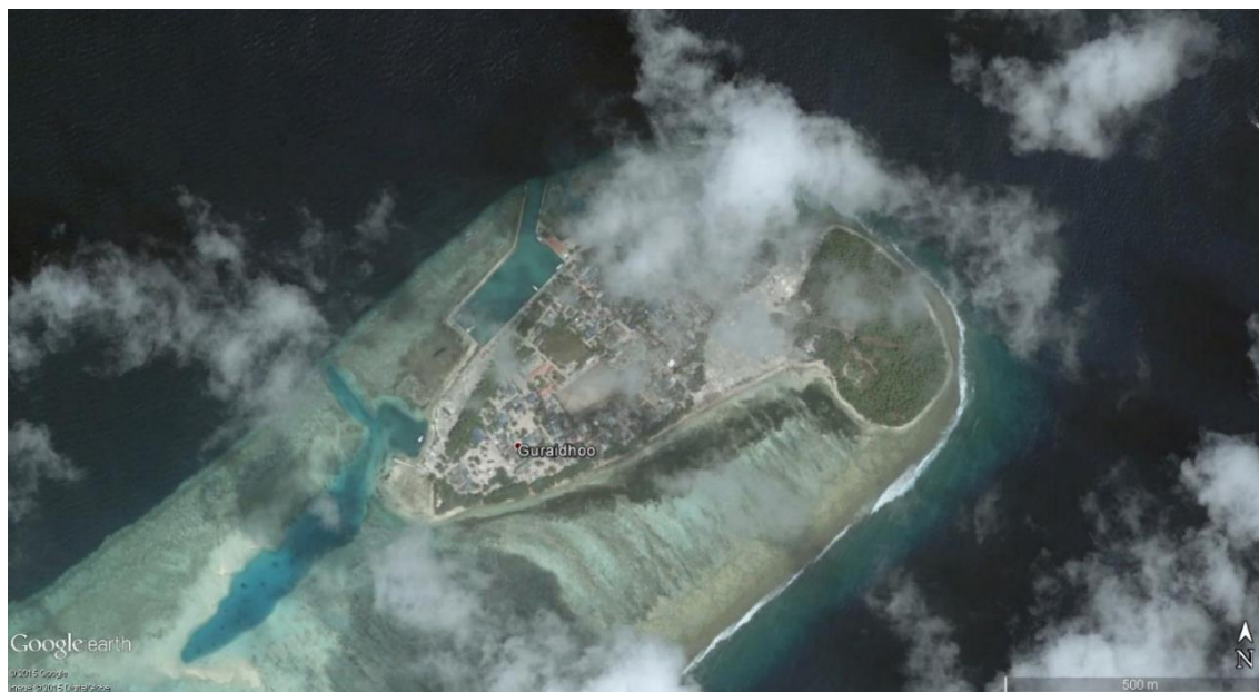
Figure 2 Location of the existing harbour
