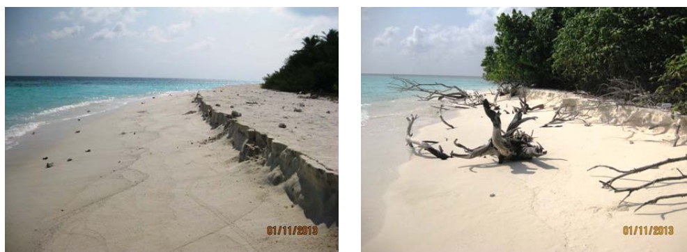
Figure 23: Erosion scarp along the north / north-eastern side was visible, and in some areas high tide mark is close or inside the vegetation line.
