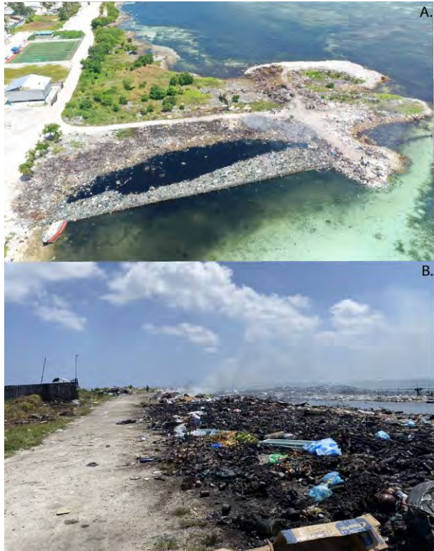
Figure 2: Photos from Maafushi. (a) Drone photo of current waste dump site (b) open burning at waste dump site
