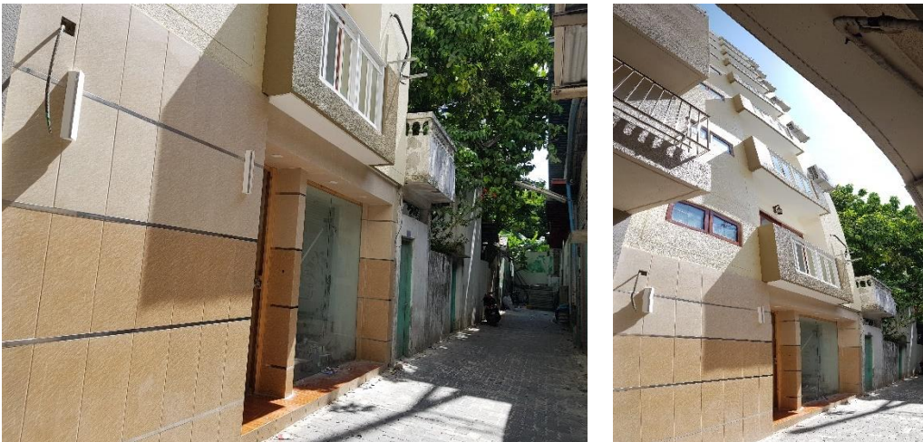
Figure 20: House adjacent to the project site under construction
