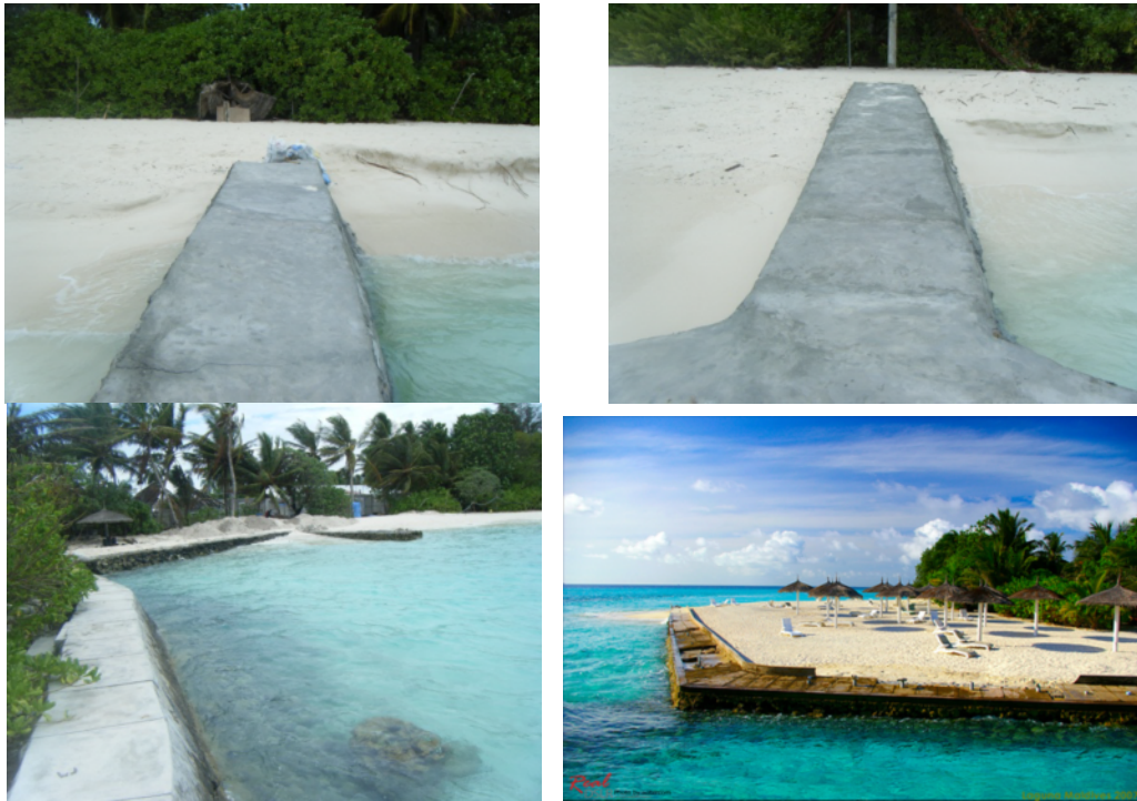
Figure 13. showing some of the coastal structures found around Laguna Island, the top two pictures shows typical impact of groynes, (erosion on one side and accretion on the opposite side). (Bottom left) is disoriented coastal structure where the groyne on the left could be eliminated. (Bottom right) picture shows the seawall constructed on the northern tip of the island to prevent erosion and protect the island.
