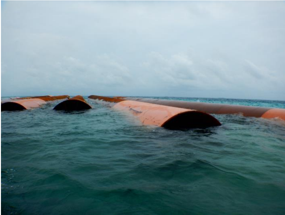
Figure 4.4: Steel pipes placed on reef flat
