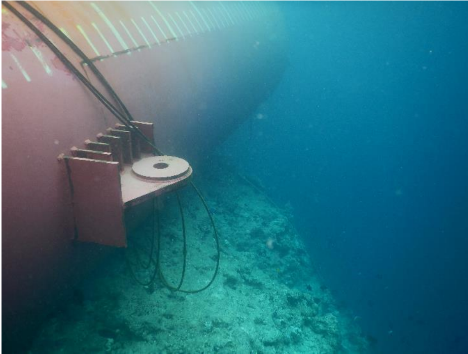
Figure 4.6: Steel pipe placed on northern side of Gulhifalhu
