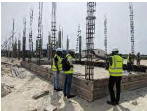
Admin Building foundation beam work
