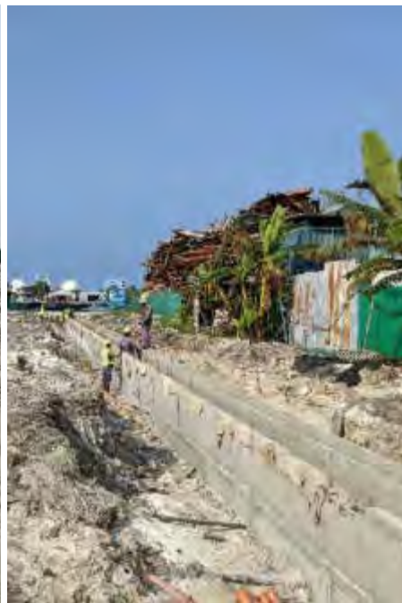
Trench-H (works on going)
