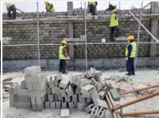
Parking shed (These unapproved blocks have been removed now)
