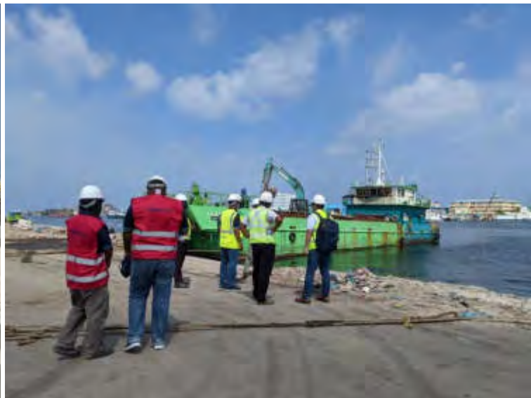
Inspecting ship ramp
