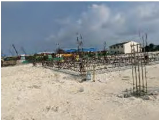
Admin Building foundation beam work
