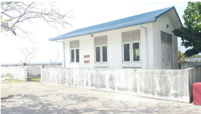
Figure 4.16 Existing RO plant facility on the island
