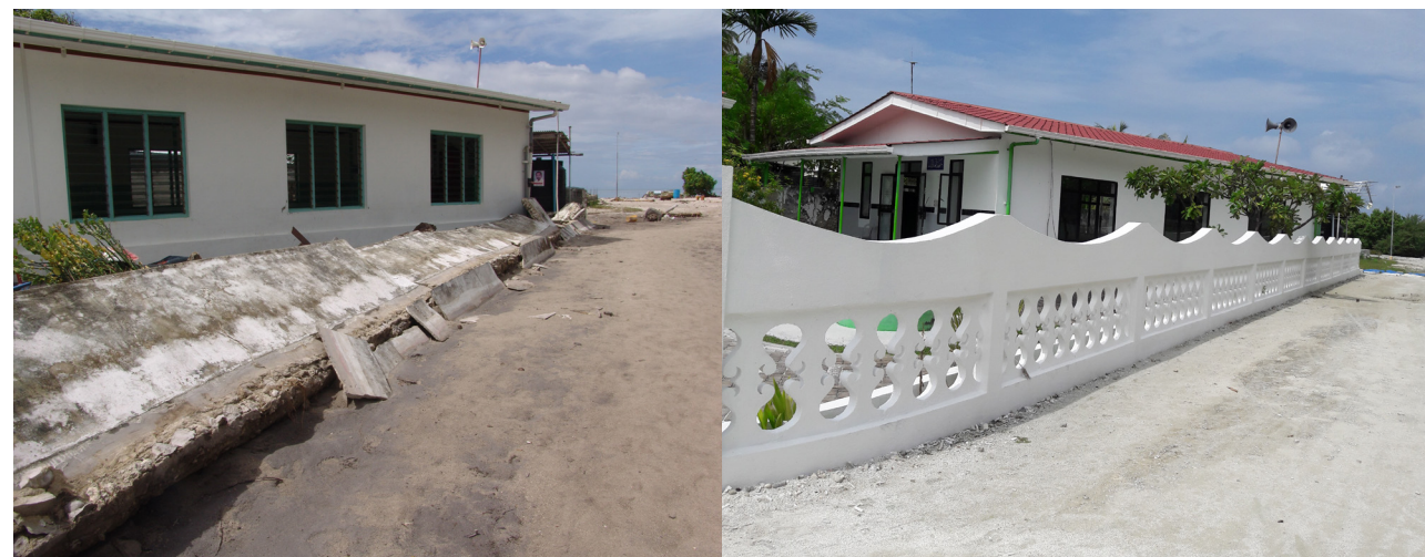
Boundary wall of this Mosque damaged during Tsunami rebuilt
