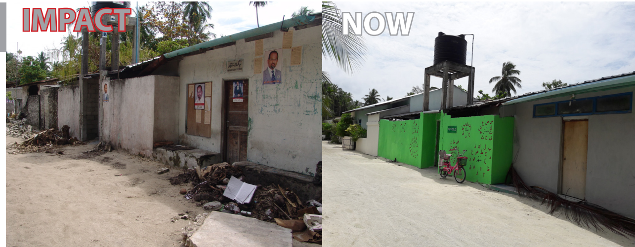
Partly damaged house renovated and used as Quran class now
