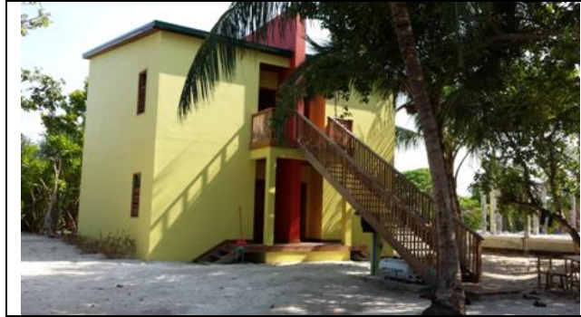
Figure 5: The mockup house constructed at the site
