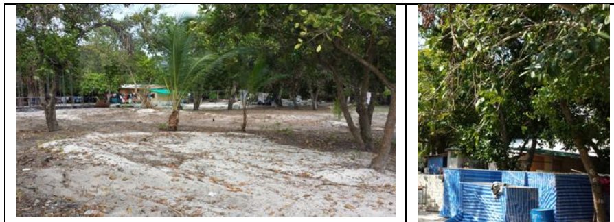
Figure 7: Temporary facilities for workers established in the land plot.
