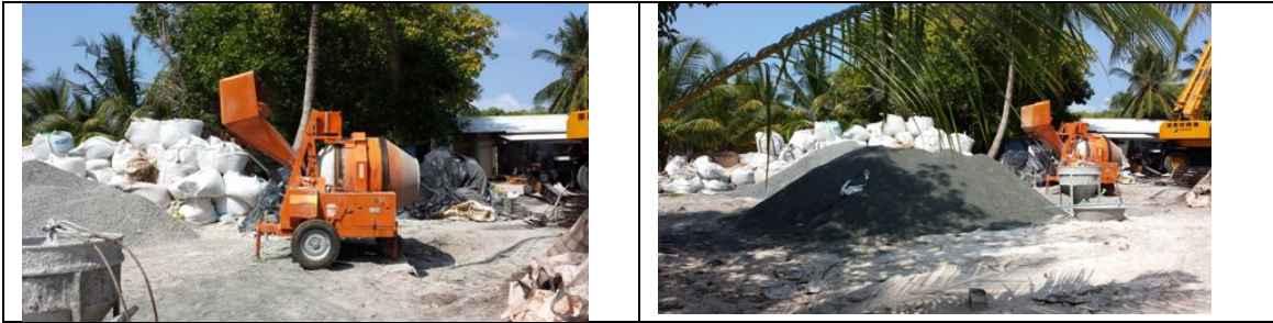
Figure 8; Construction material and equipment mobilized in the site
