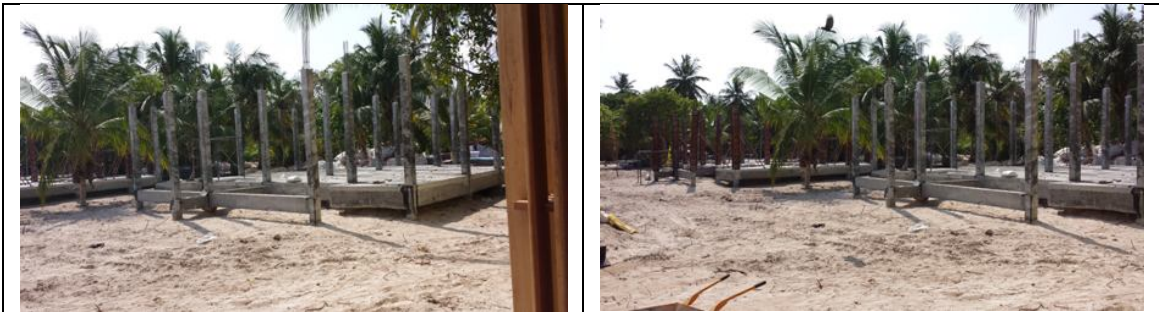
Figure 6; Foundation work for two more rooms started
