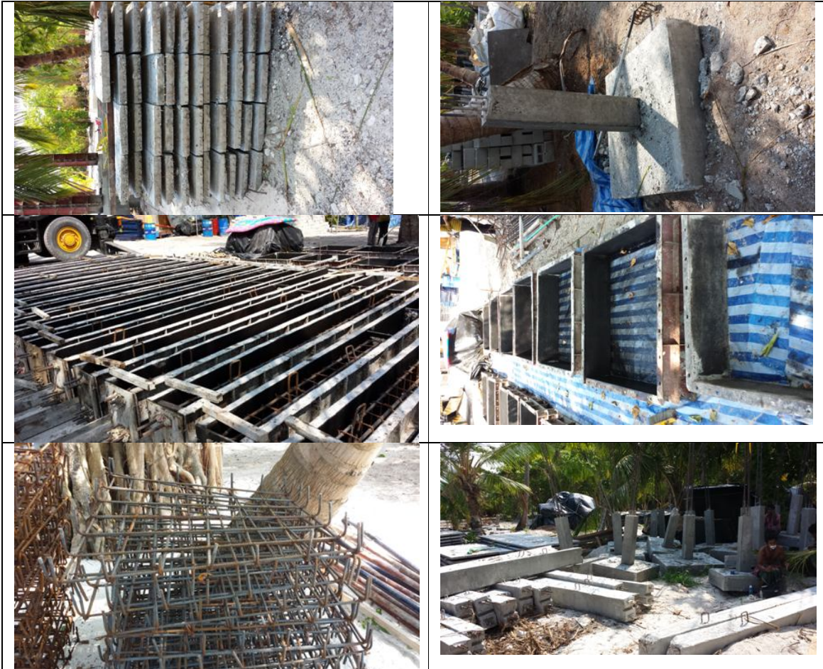
Figure 9: Precast concrete beams, pads and sheet production at the site.
