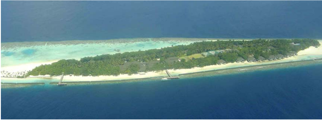
Figure 10: Aerial view of Lily Beach after the breakwaters were constructed.
