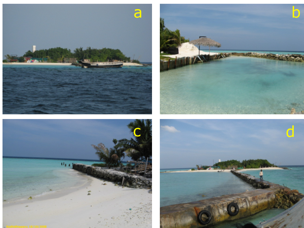
Figure 10: Existing coastal structures on the island, Island as seen from a distance (a); fish pond (b), breakwater going to south (c) and main T-breakwater facing east (d).
