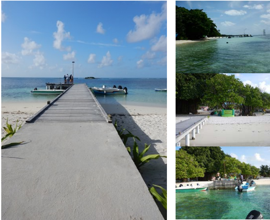
Figure 2: Existing Jetty B. Fehendhoo northern side
