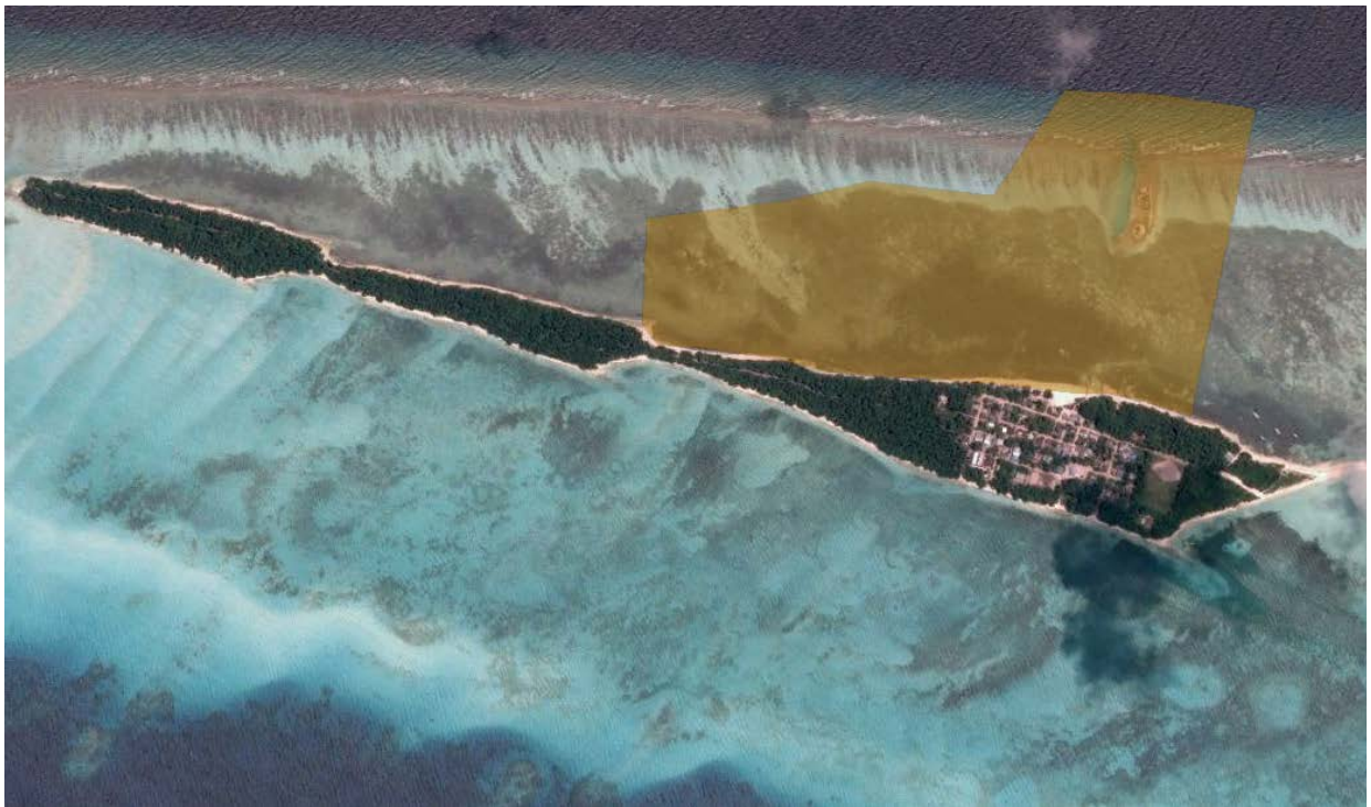
Figure 8: B. Fehendhoo island access and Jetty construction project study area
