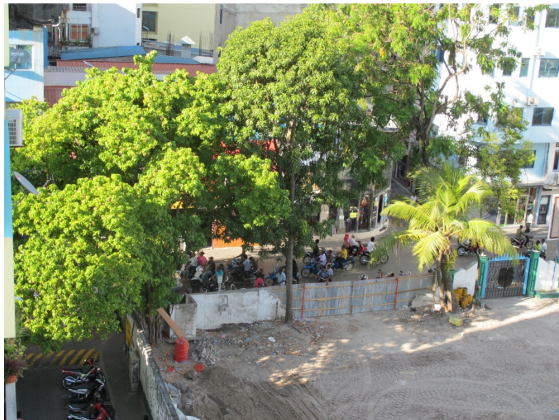
Figure 2: Existing condition of the project site.
