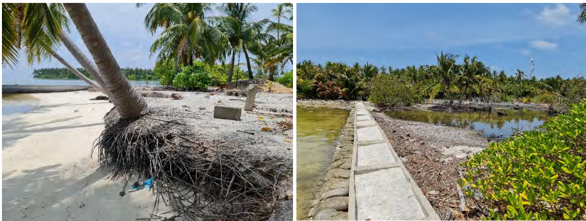
Figure 17. South eastern corner area
