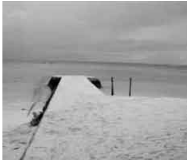
Groyne in Alimathaa, V. Atoll
