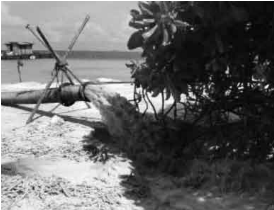
Beach nourishment at Velidhoo, North Ari Atoll
