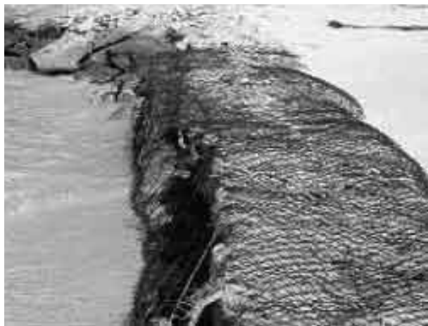
Gabions in a seawall at North Ari Gangehi
