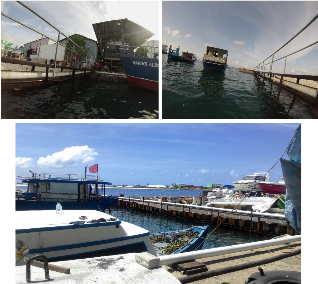
Figure 20: existing jetty at Hawks Thilafushi site
