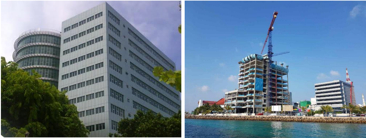
Figure 7: The 14 Storey Velaanaage Office Complex (left) and ongoing 25 Storey IGMH Building
