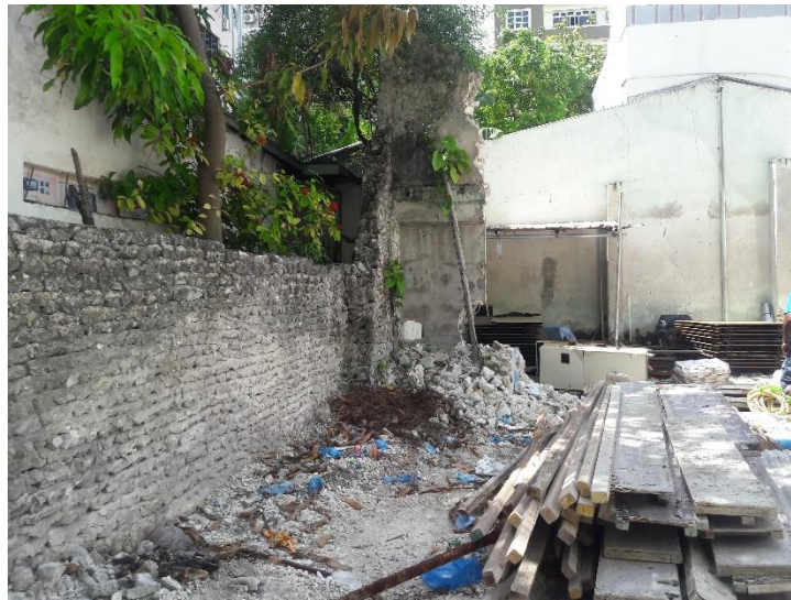
Figure 10: Temporary setting works within the plot
