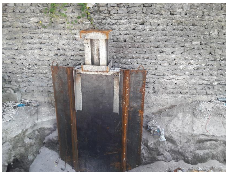
Figure 11: A sample sheet pile done to test protection of adjacent buildings
