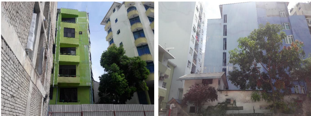
Figure 38: Multistrey buildings found on the opposite side of the plot
