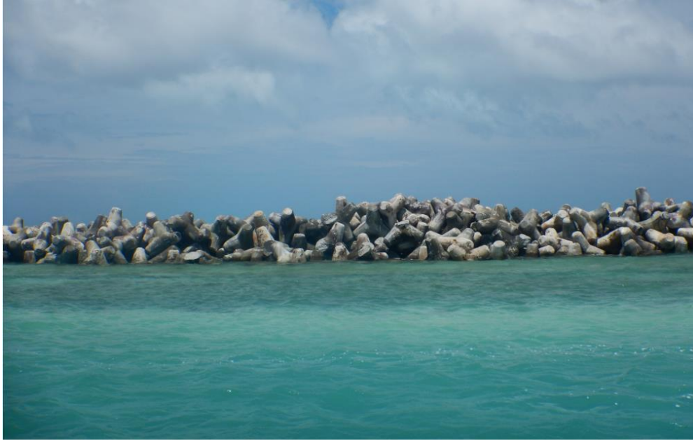
Figure 92: Tetrapod concrete armour units offshore breakwater in Male'
