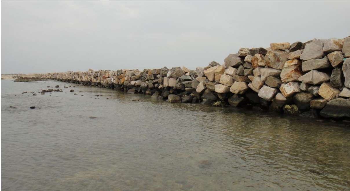
Figure 91: Example of offshore breakwater constructed at Maamigilli Island
