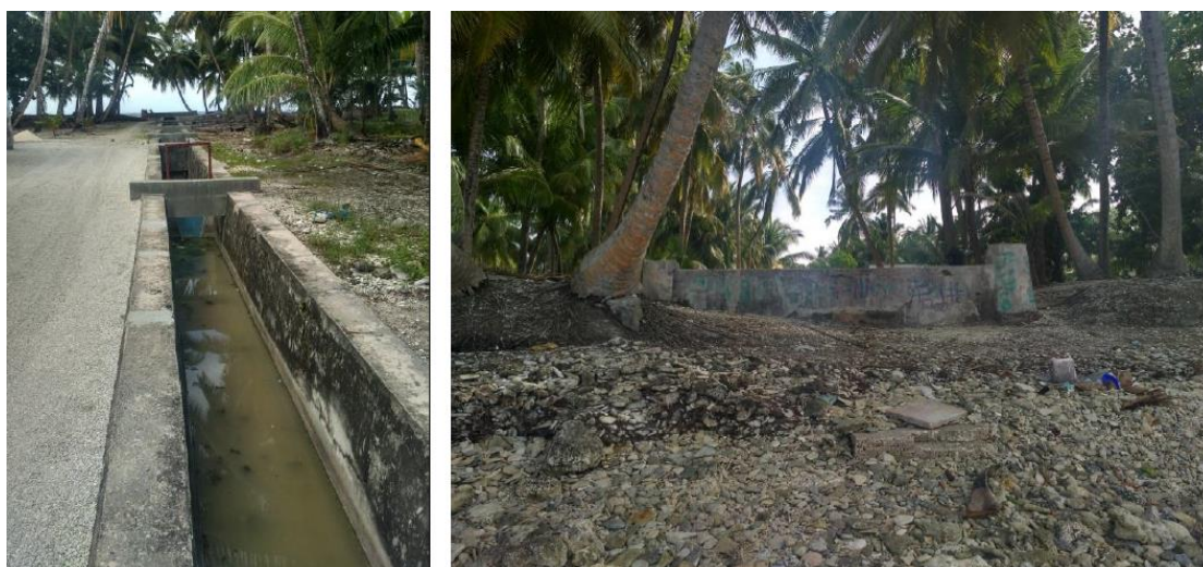
Figure 103: Existing drainage channel (left) and location of outfall towards sea intersecting proposed revetment (Source: RHDHV, 2016)
