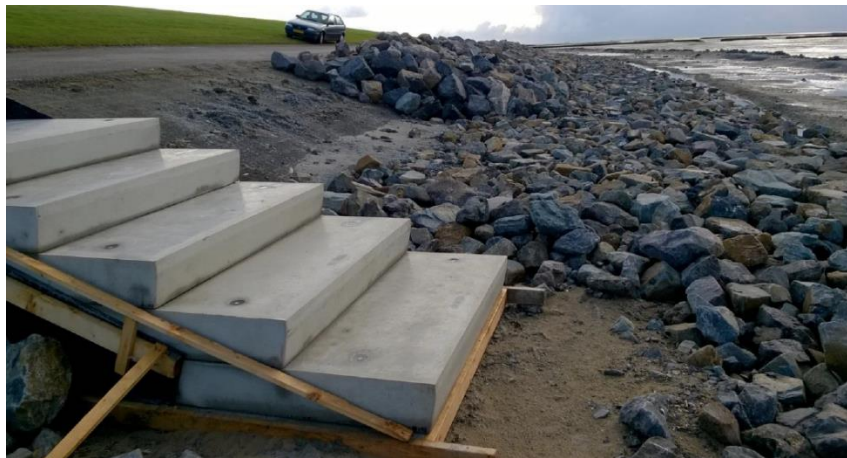
Figure 102: Example of concrete steps in a rock armour revetment (isle of Ameland in the Netherlands), Source: RHDHV, 2016
