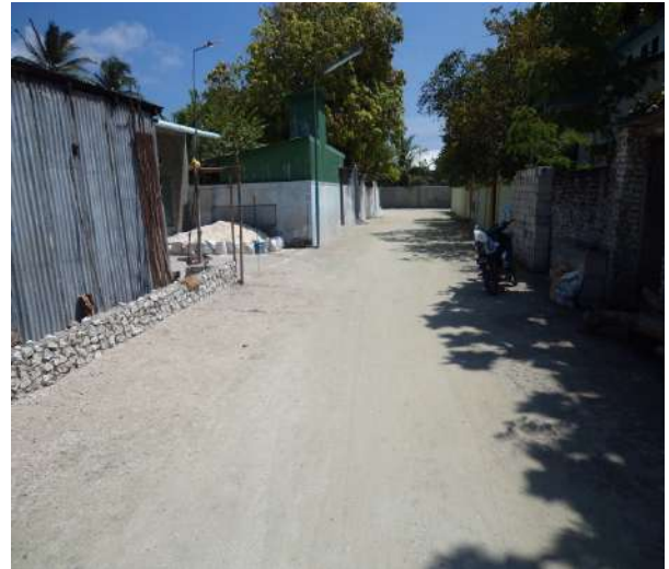
Lowest point flooding is taking place
