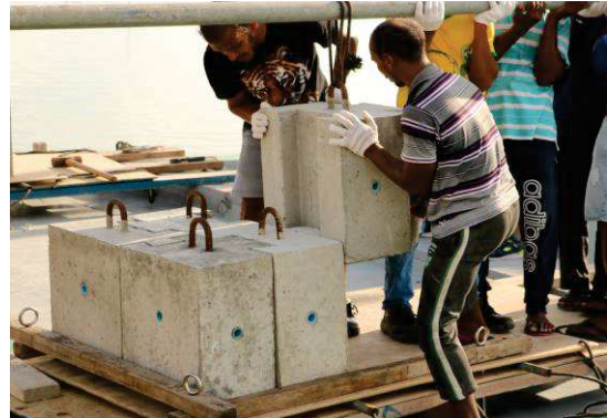
Figure 2.8: Concrete anchor block assembled on the vessel for deployment.
