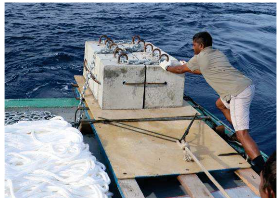
Figure 2.10: Both anchor blocks resting on the deck of the vessel is simultaneously pushed into the sea.
