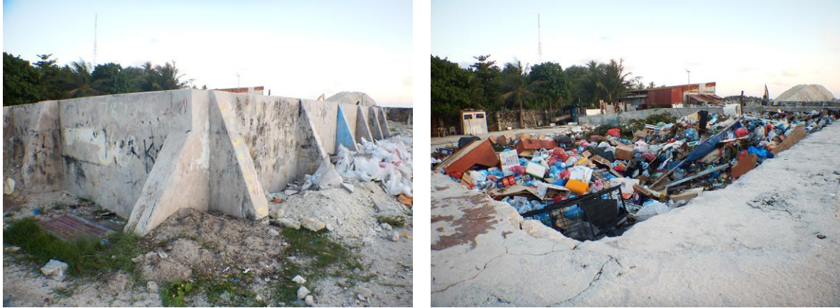
Figure 37: Waste collection yard in Villingili
