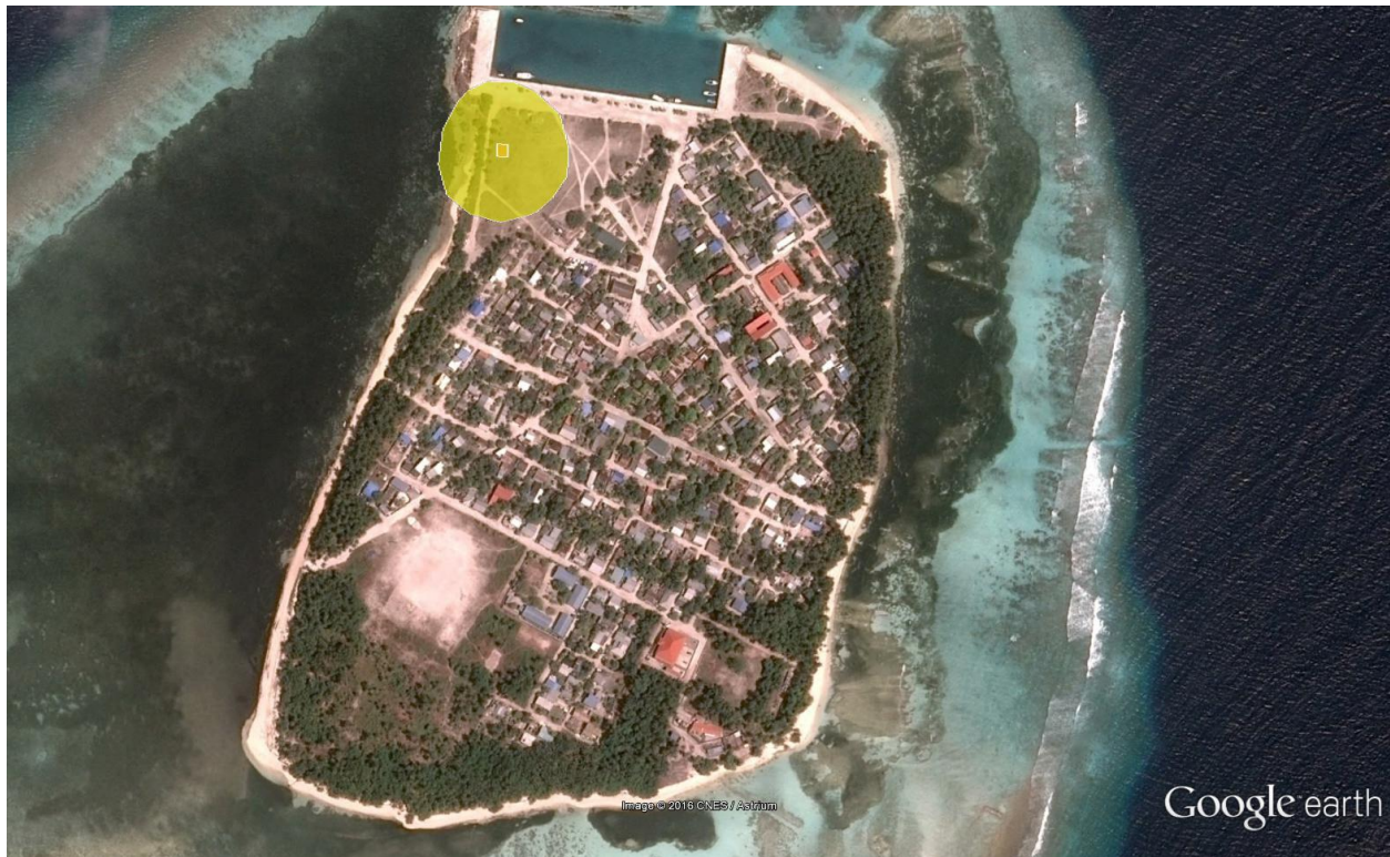
Figure 20: impact zone during construction. Orange; is primary impact zone and yellow; is secondary impact zone
