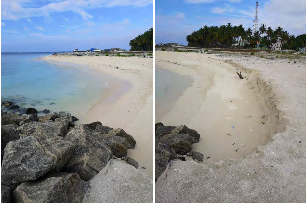
Figure 20 Erosion areas in B. Eydhafushi
