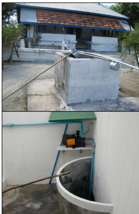
Figure 8.10: Containers connected to a long stick (locally knows as dhaani ) and electrical pumps (bottom photo) are commonly used for extracting groundwater from wells. Bottom photo taken from MWSA (2005).
