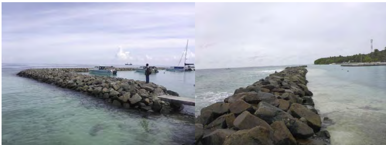
Figure 4.10 Current break water design for harbours – Raised rock boulder breakwater in Rasdhoo and Maalhos
