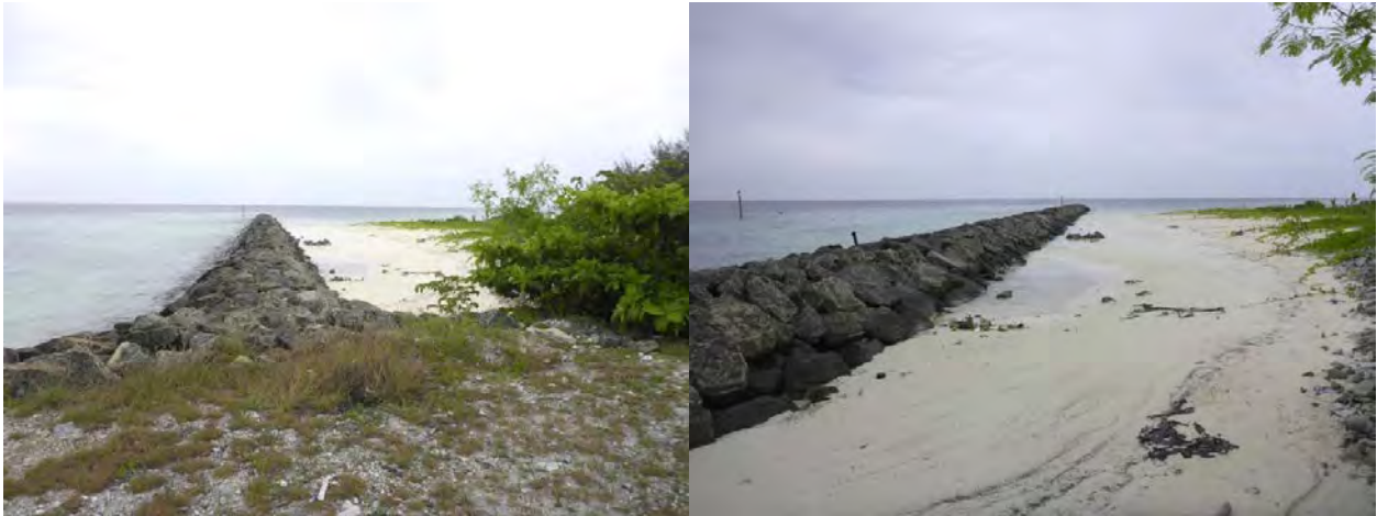
Figure 4.13 Groyne constructed in Feridhoo to prevent sedimentation in harbor basin and to prevent erosion
